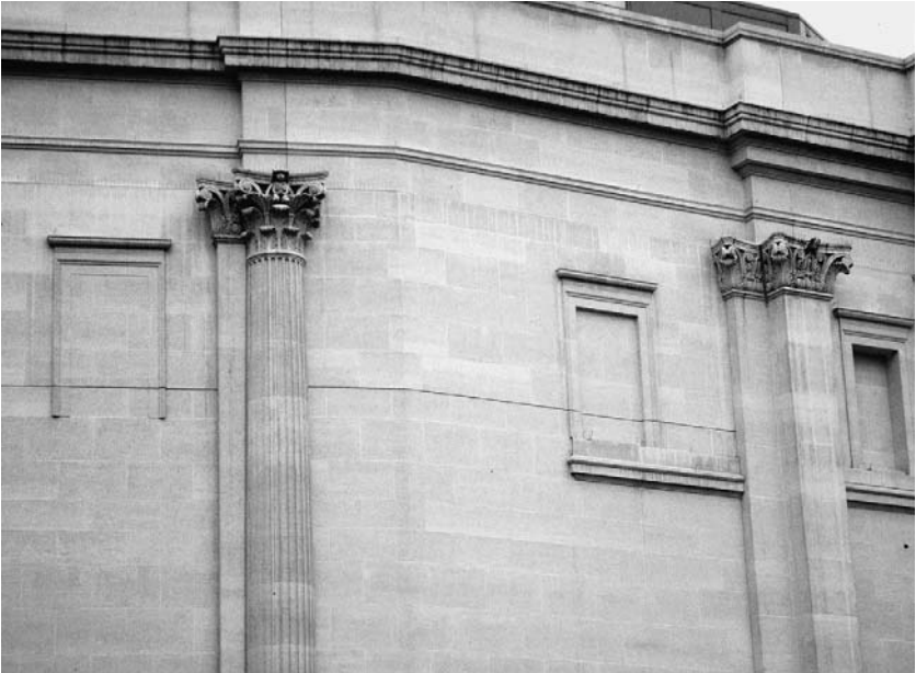
4.6 The Sainsbury Wing of the National Gallery in London, designed by Robert Venturi. Here a kind of architectural joke is played in which the rules of the original Wilkins Building are followed slavishly at first, and then progressively ignored as we move further away
