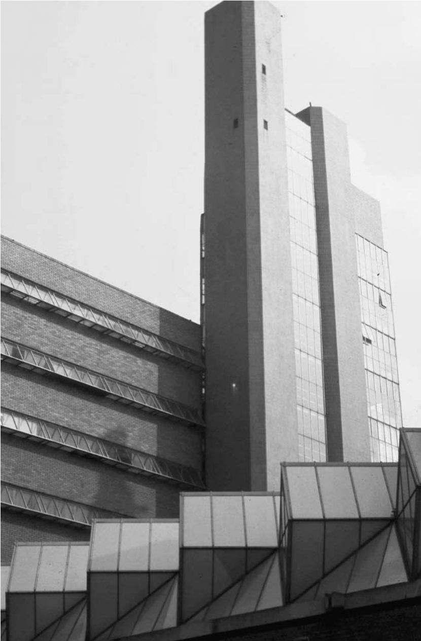
4.12 The Engineering Faculty Building at Leicester University by James Stirling. Both formal and symbolic language is clearly in evidence here. A form free of classical rules is nevertheless heavily redundant and rule-bound. The machine-like shapes also suggest the activities it contains and the professions to which its students aspire
